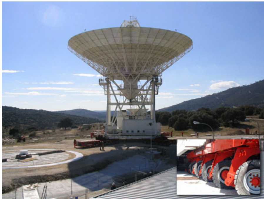
Caption: Giant Deep Space Network antenna in Madrid is moved using four 12-axle, 24-wheel crawlers.
